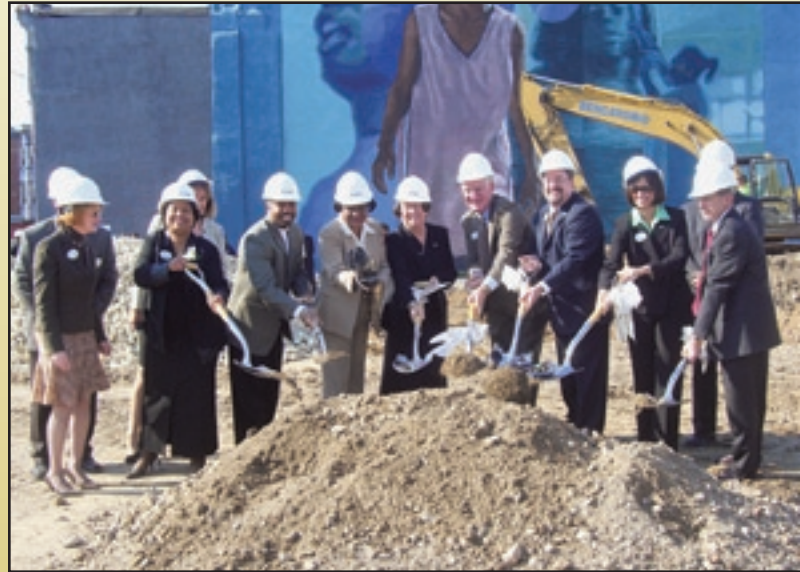
Digging In: Presby leadership joins Philadelphia City Councilwoman, Jannie Blackwell, in celebration of the groundbreaking of a new affordable housing community at 34th and Haverford in Mantua.
